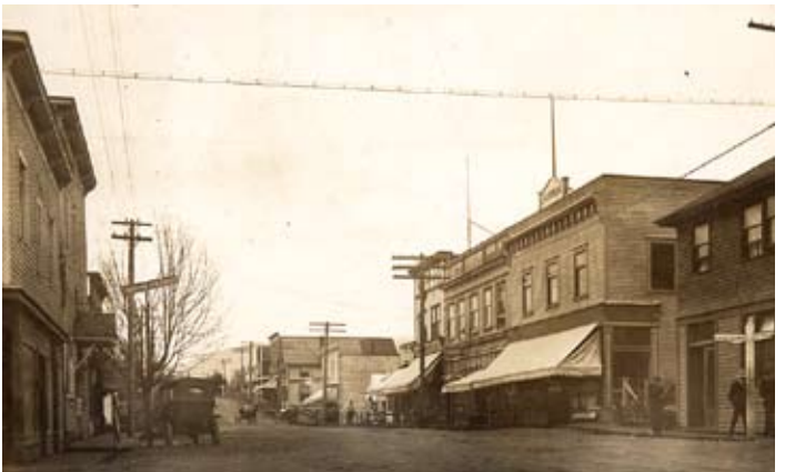
Courtenay before the fire
